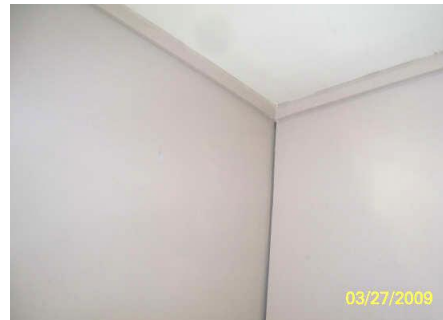
After air sealing. Substantial gaps in plywood seams sealed to prevent air leakage through thermal boundary
