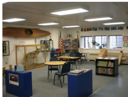
4-lamp fixtures de-lamped to three 25 watt T-8 lamps each for additional savings.
