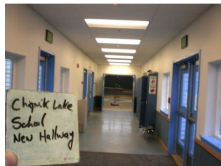
New school addition re-lamped with 25 watt T-8 lamps.
