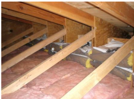
Existing R-19 fiber glass attic insulation placed between ceiling joists on 24 inch centers.
