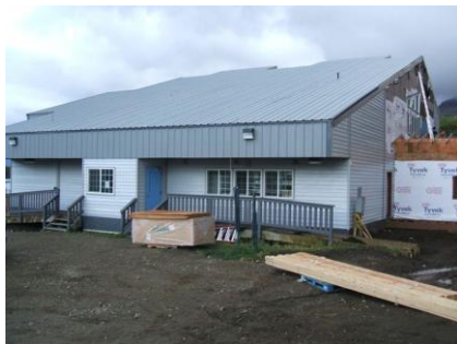
New addition being added to old school building.
