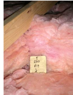
New R-30 fiberglass bats installed on top of existing R-19 insulation.
